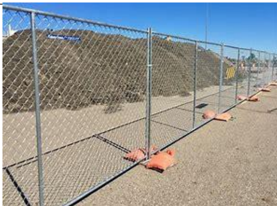
Temporary site fencing
