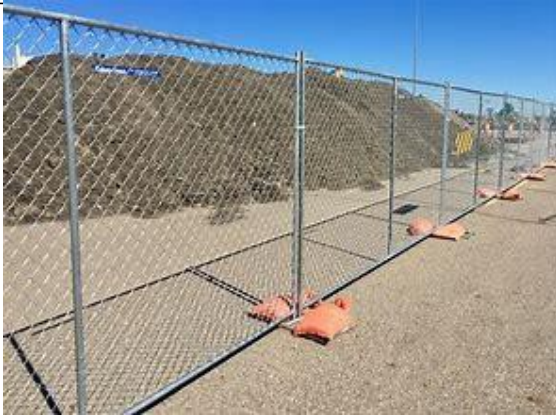
Temporary site fencing
